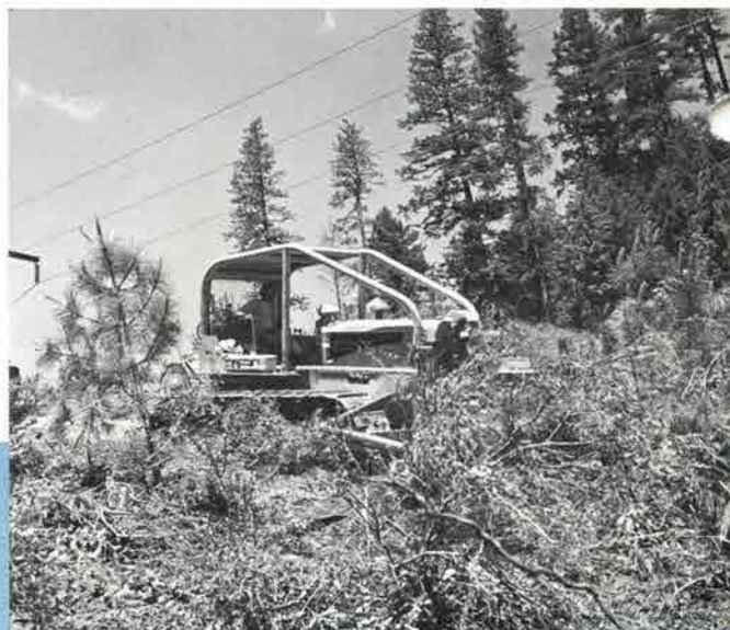
Clearing out the growth on right-of-way of power transmission lines. Utility companies have drastically cut these clearing costs and greatly increased production.
