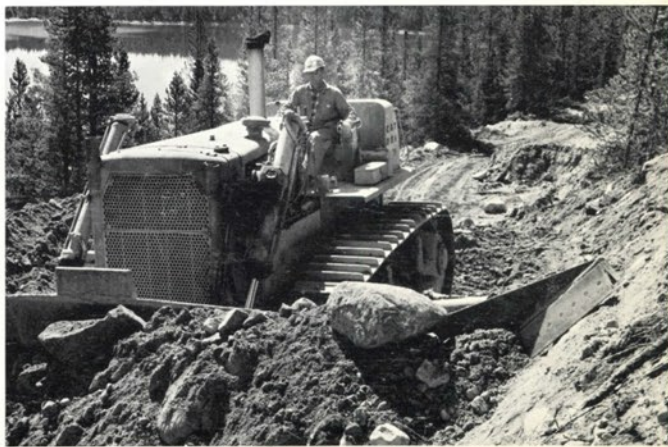
SLOPER BLADE cutting a slope 2 miles above sea level high in the Colorado Rockies. Note the boulders and rugged material. Cutting this slope was another routine operation saving the contractor many hours and operating costs.
