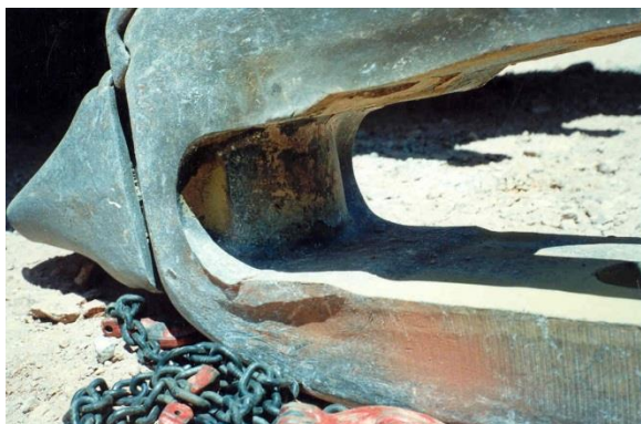
14 Months... The same CPS-10 bucket lip stabilizer unit and CPS-10 base adapter after 13.2 million tons of material has been removed.
